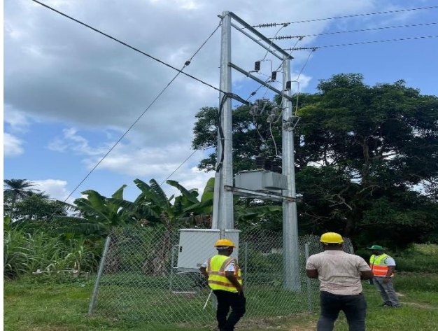
Contractor (Wilkins Engineering) inspecting the completed auto-recloser installation.
